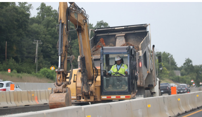
Widening between exit 137 and exit 141
