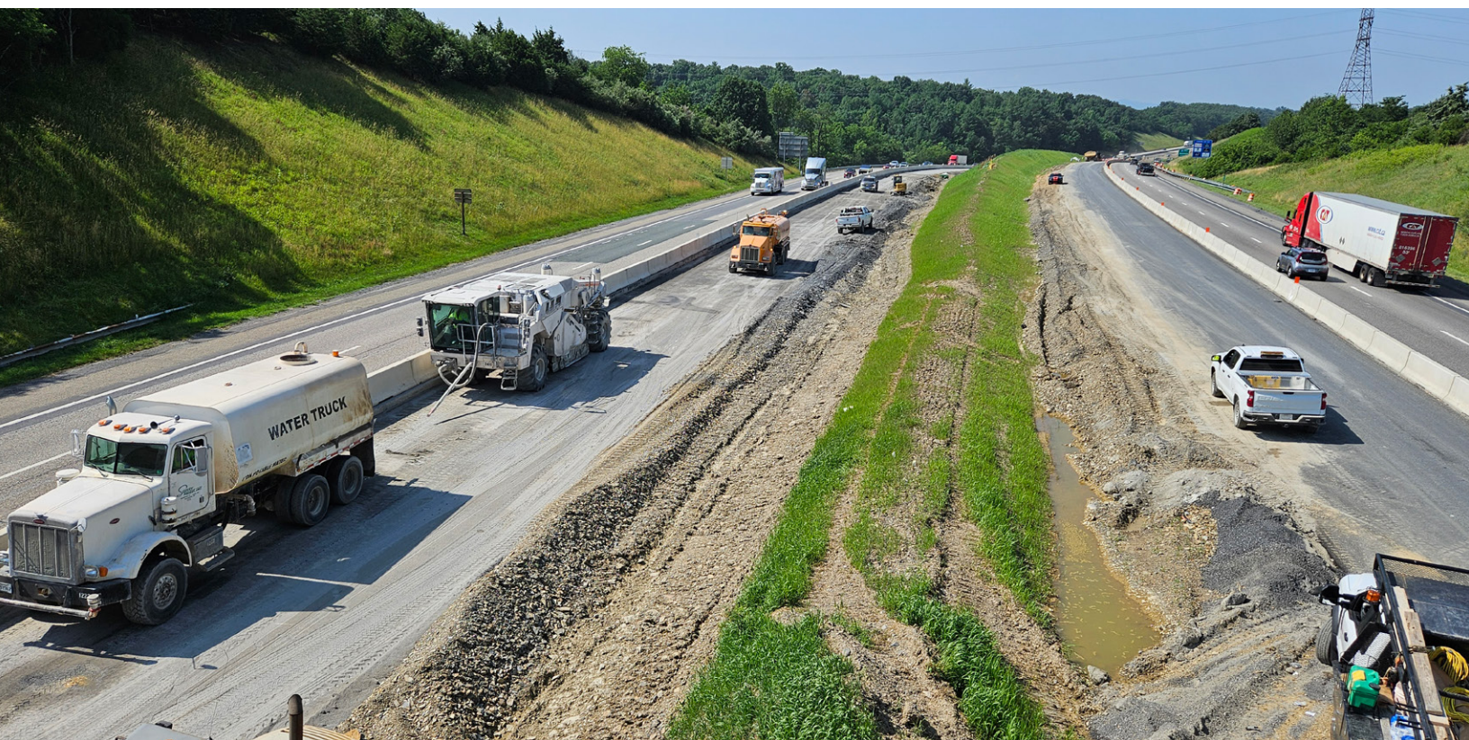
Grading and paving work for I-81 widening near Staunton
