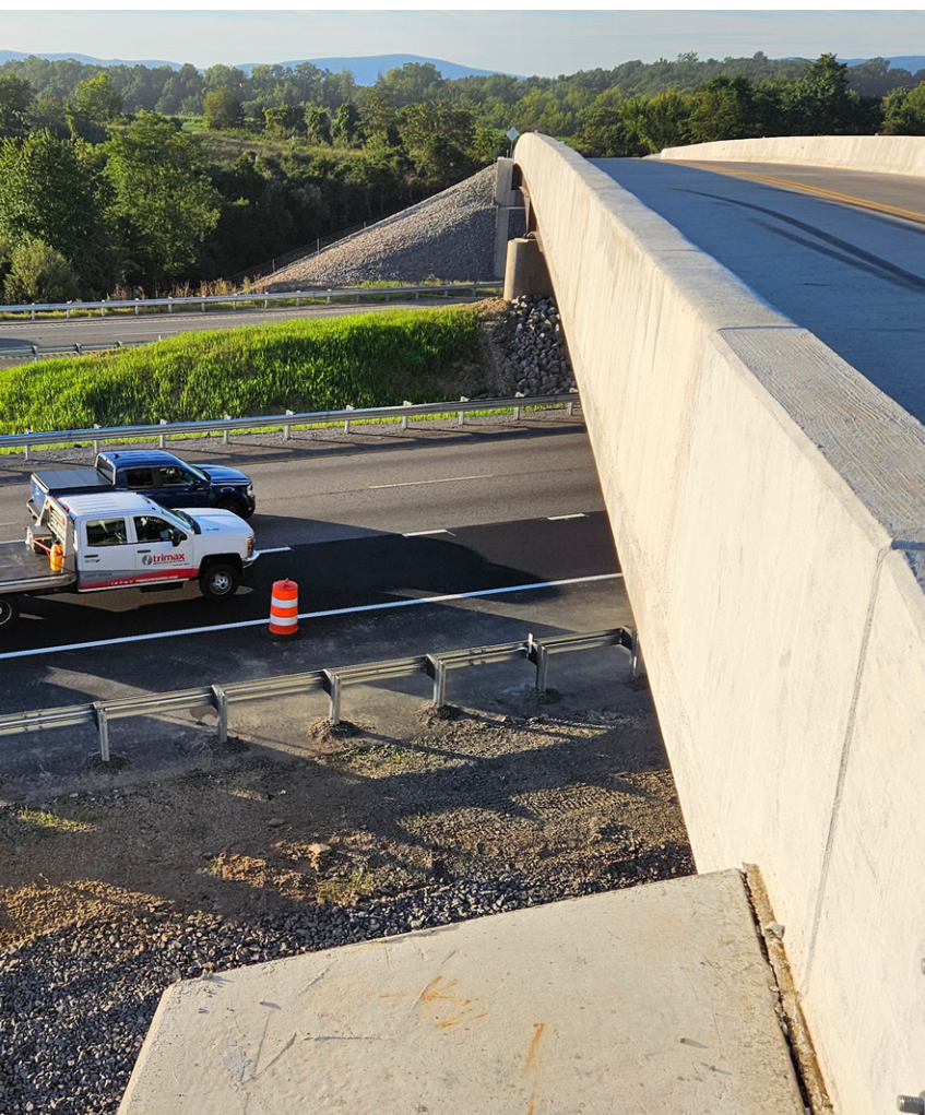
Southbound I-81 auxiliary lane open
