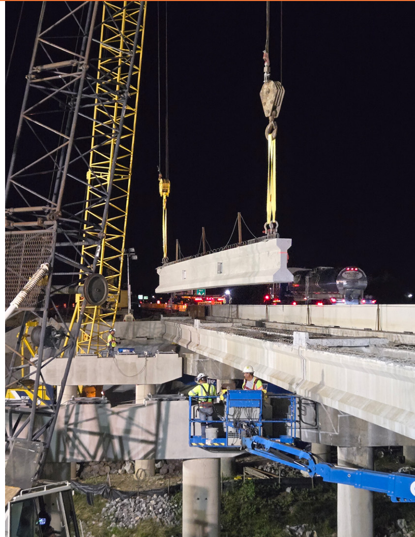
Bridge girder placement near Staunton
