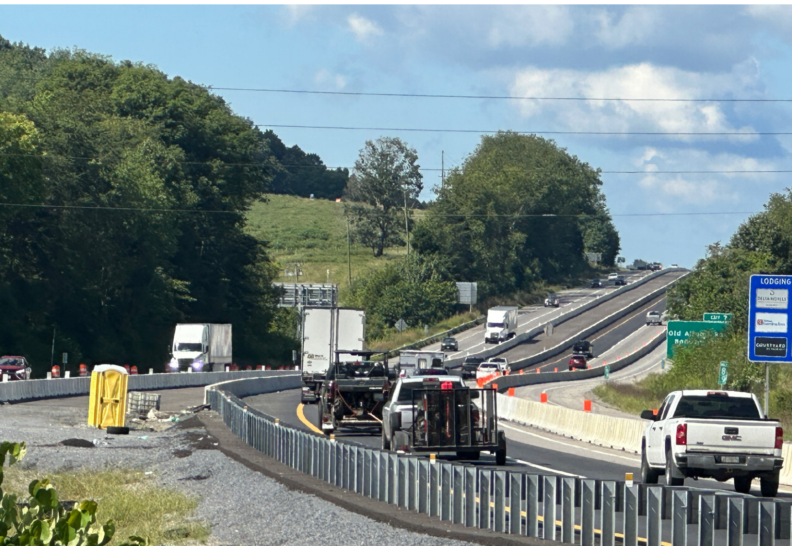
Widening I-81 southbound from exit 10 to exit 7
