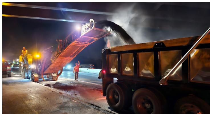
Final milling and paving for new I-81 auxiliary lane
