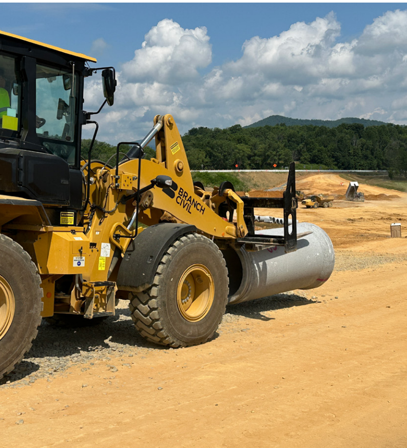
Grading and drainage work at I-77 exit 41
