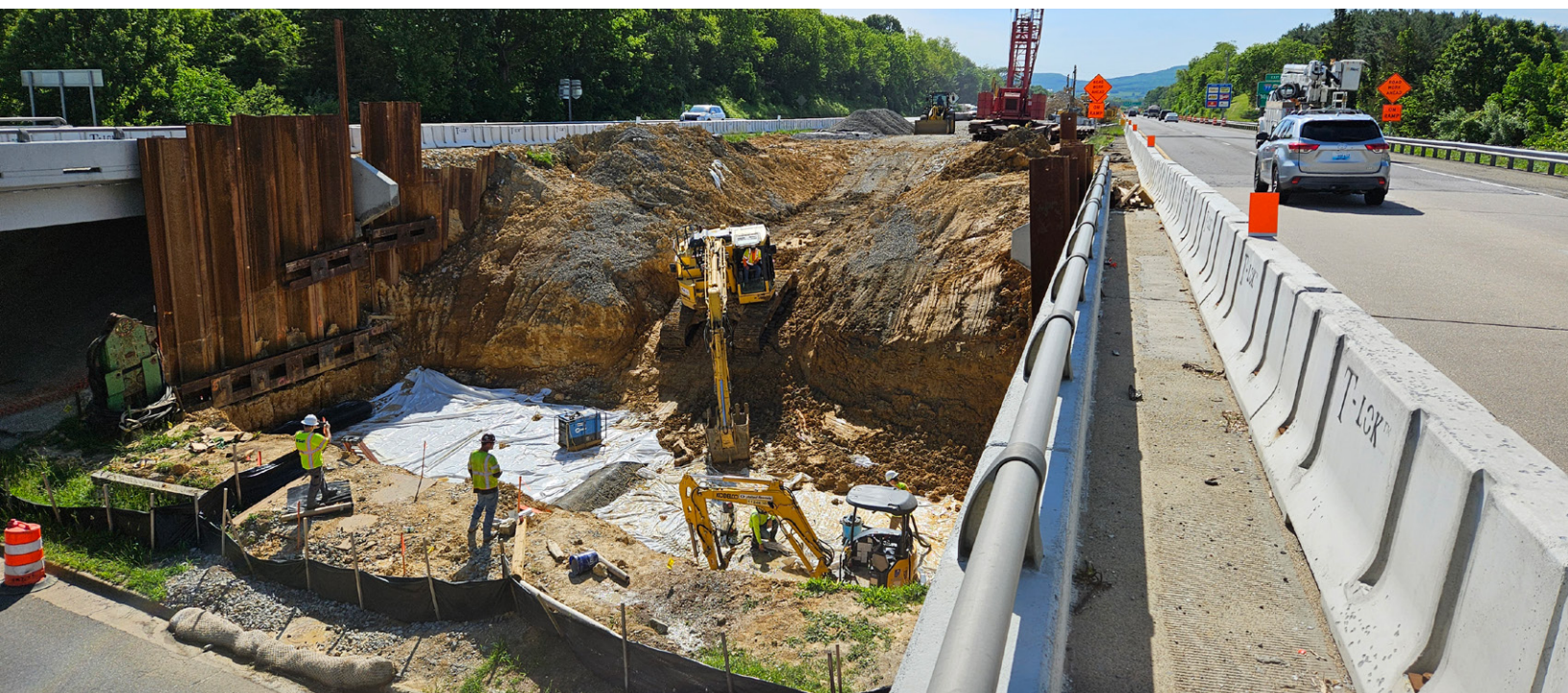
Early-stage construction work on I-81 bridges over Peppers Ferry Road near Wytheville
