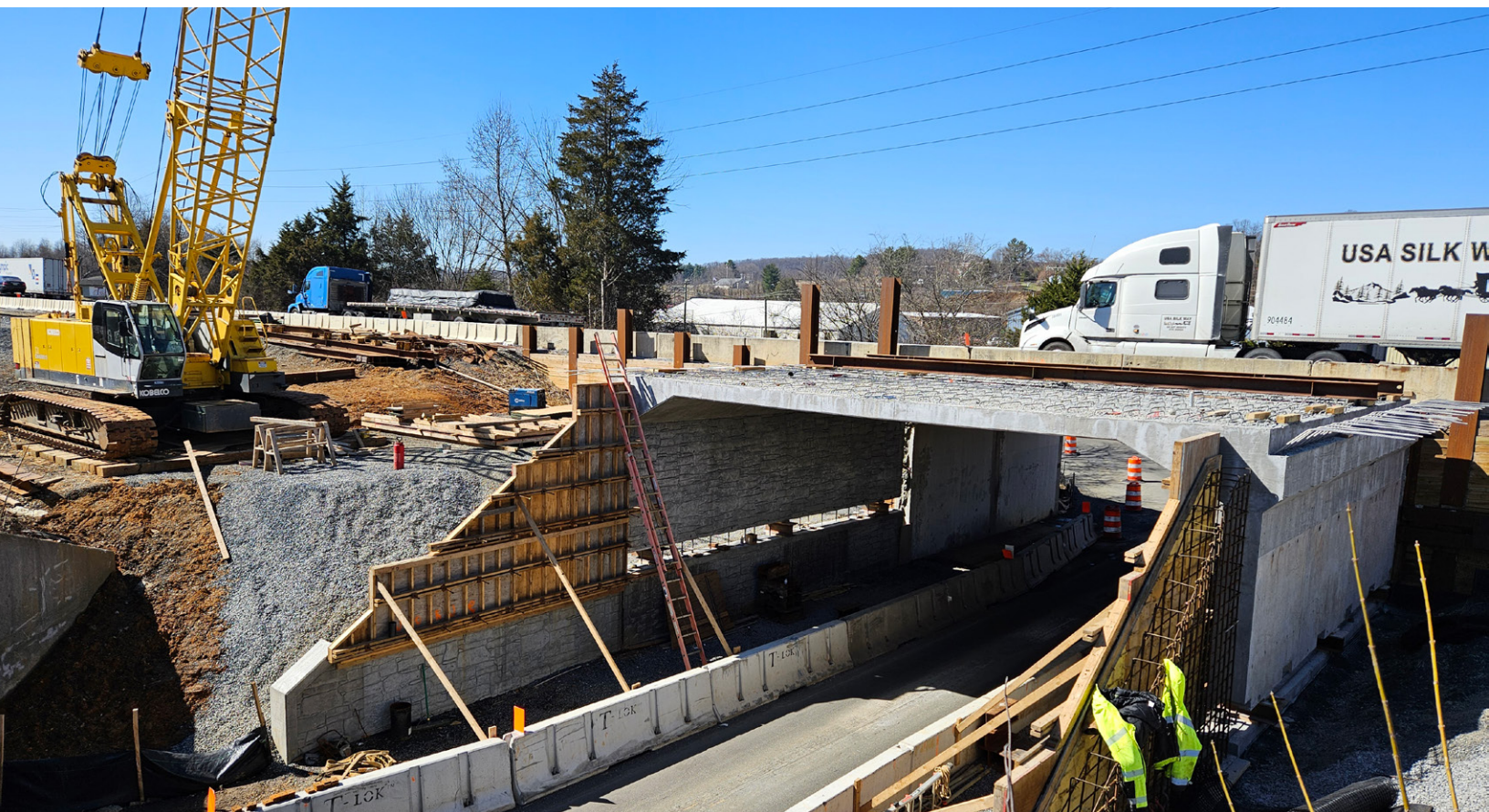
Bridge work on I-81 over Old Dominion Road near Bristol
