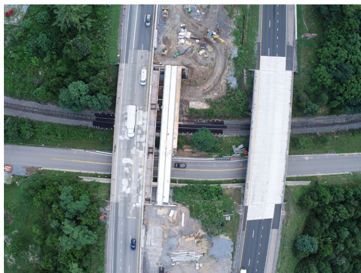
Bridge widening for Staunton-area I-81 project
