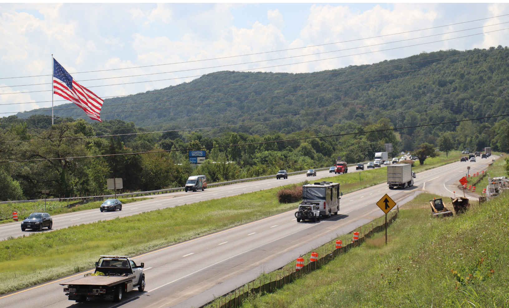
Early phases of I-81 widening project between exit 143 and exit 150
