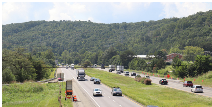
Widening between exit 143 and exit 150
