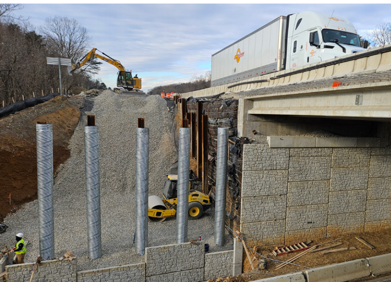
Bridge construction near Salem
