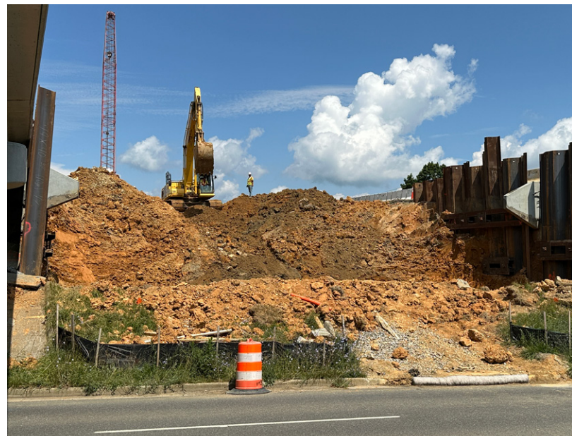
I-81 bridge work at Peppers Ferry Road
