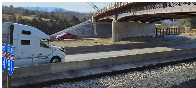
Construction of Route 635 bridge over I-81 in Augusta County
