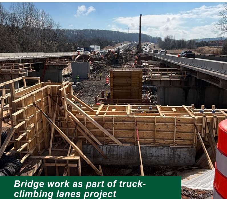
Replacement of Cedar Creek bridge on southbound I-81
