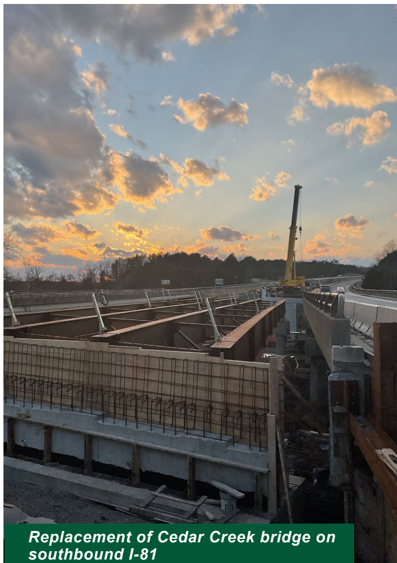
Steel bridge beams in place over Cedar Creek near Strasburg
