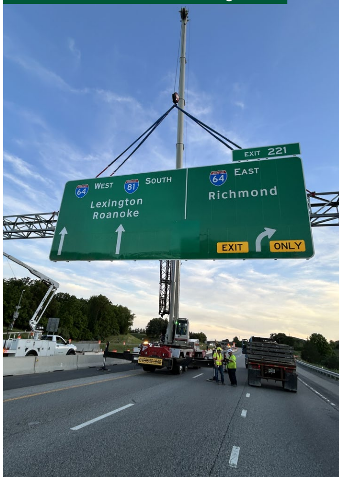
Temporary I-81 South closure allowed installation of new overhead signs
