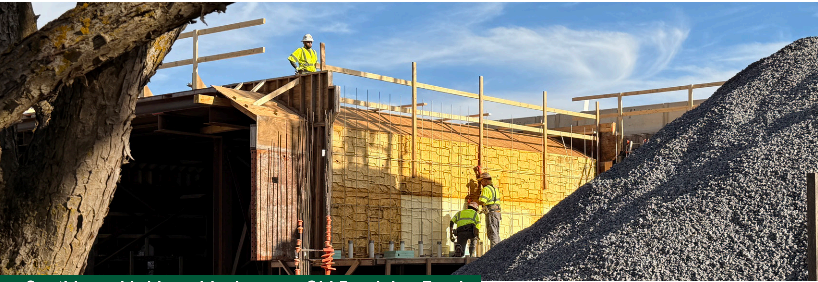
Southbound bridge widening over Old Dominion Road
