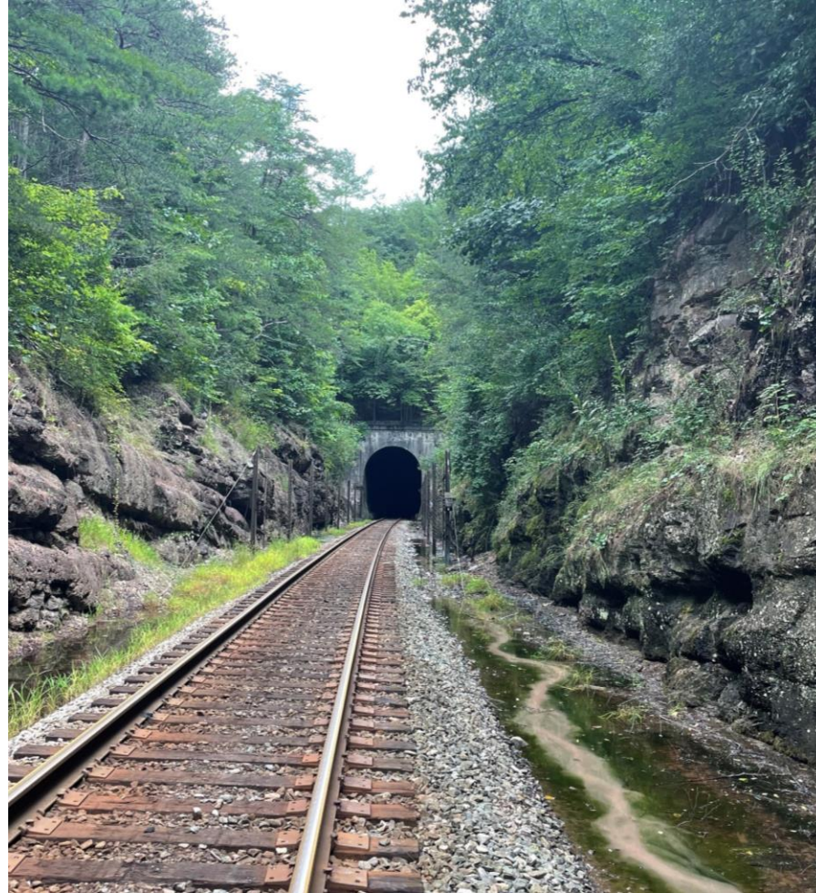
Slate Hill Tunnel
